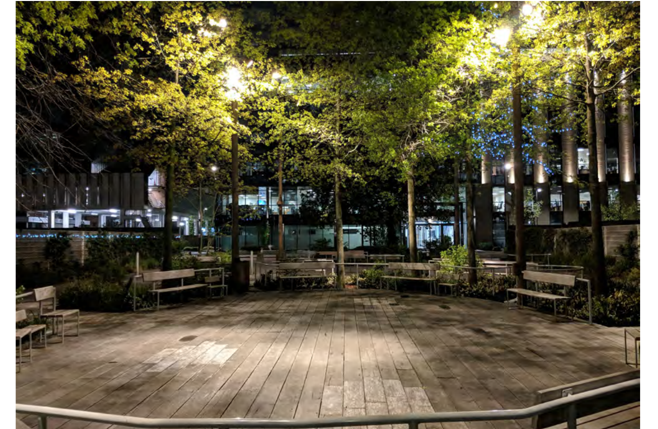
New column-mounted spotlights to the approach from Western Road creates a welcoming place after dark.
