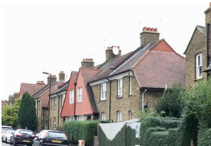
Wateville Road (east side)
