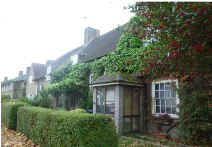
Modern porch additions
