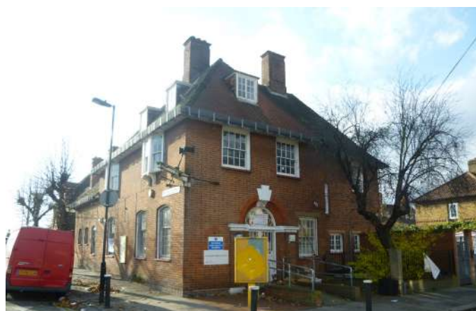
Former community hall, Tower Gardens Road
