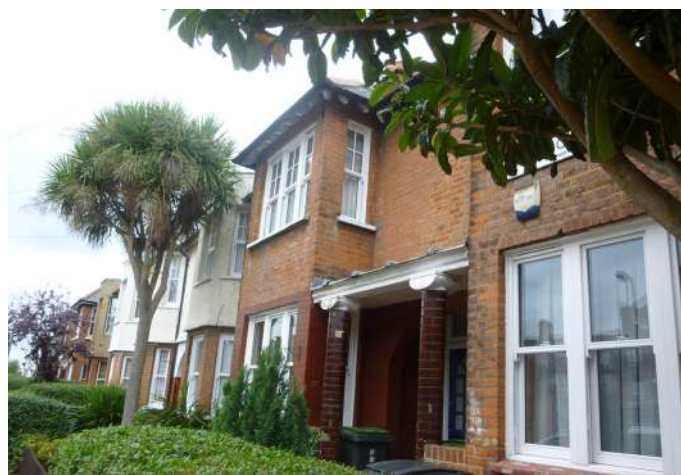
Tower Gardens Road (north side)
