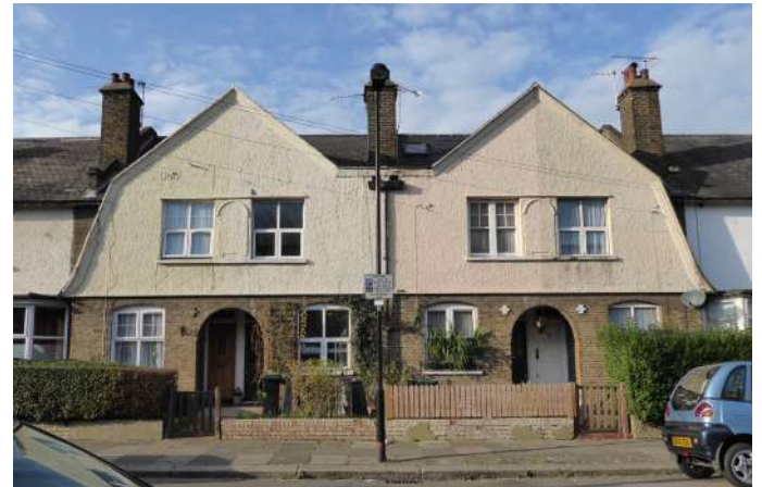
Shobden Road (west side); paired gables
