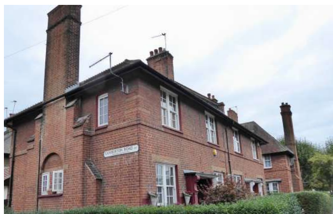
Risley Avenue (south side)
