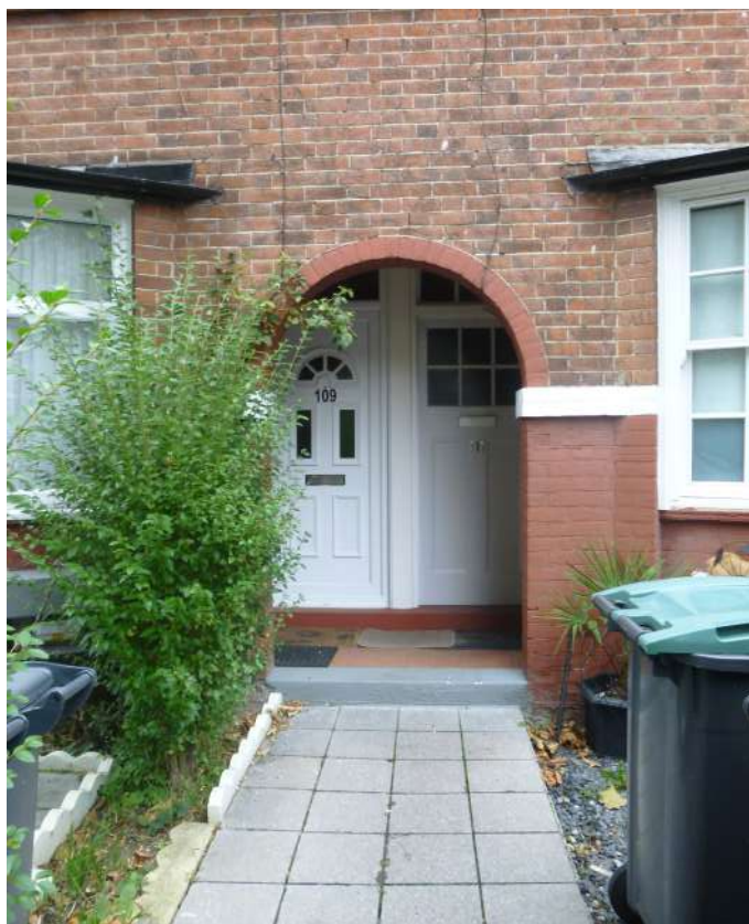
Replacement door (left) original door (right)
