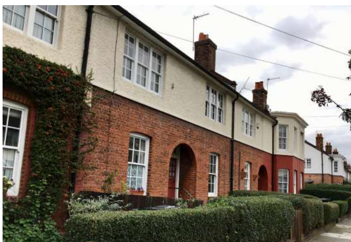
Tower Gardens Road (north side)
