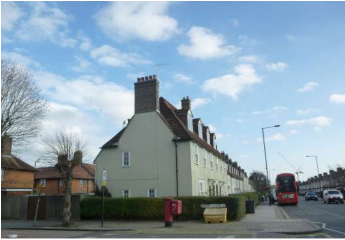
Lordship Lane: cottage flats
