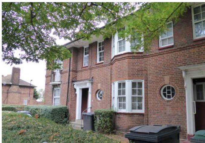
De Quincey Road (west side)
