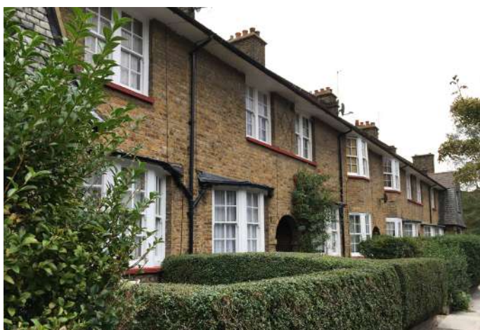
Tower Gardens Road (north side)
