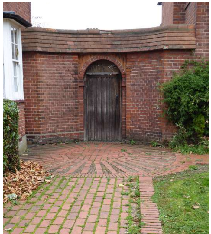
Original brick pavers
