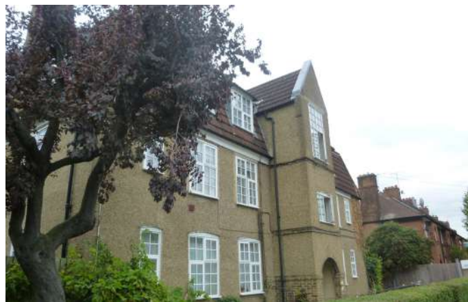
Topham Square: Risley Avenue elevation
