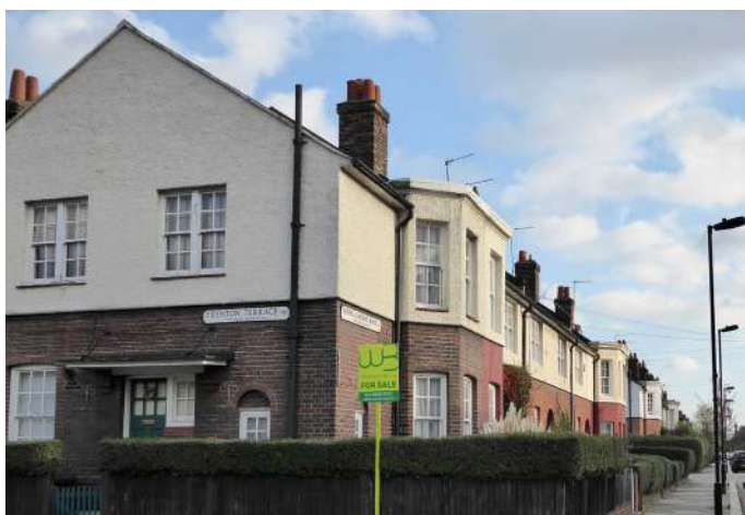
Tower Gardens Road (north side)
