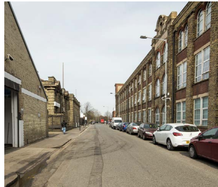
Ashley Road South © Allies and Morrison Architects
