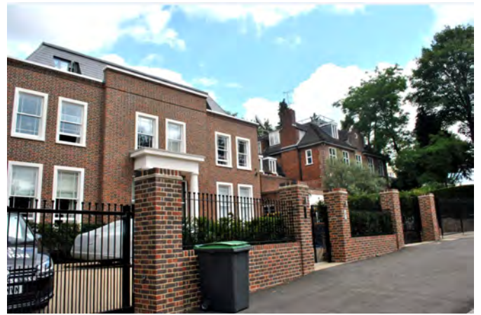
No 28 Hampstead Lane
