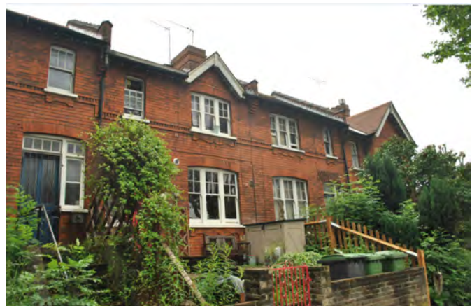
Details of the facade, North Hill
