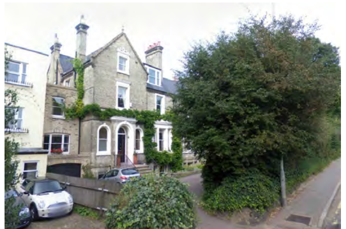
No 20 Hampstead Lane
