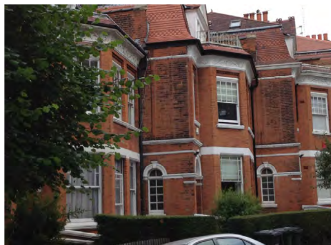
Recessed terraces, 17-19 Hornsey Lane Gardens
