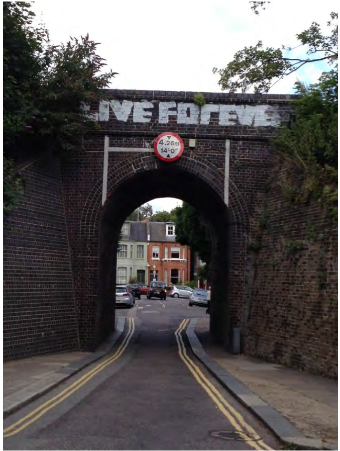
Railway arch, Northwood Road
