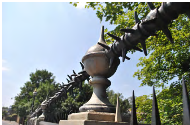
Hornsey Bridge, details
