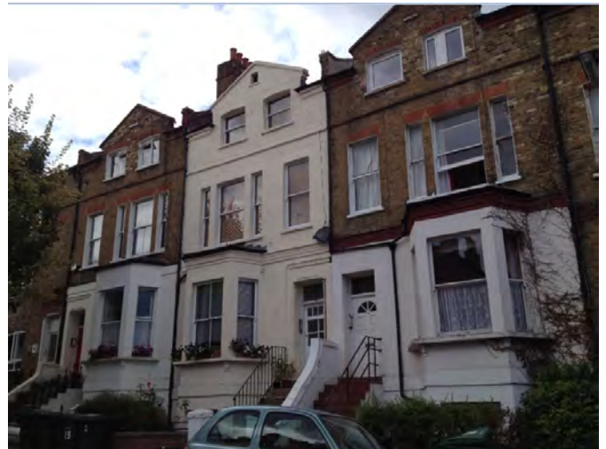
Nos 17-19 Northwood Road
