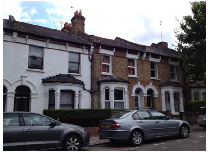
Nos 46-42, Northwood Road
