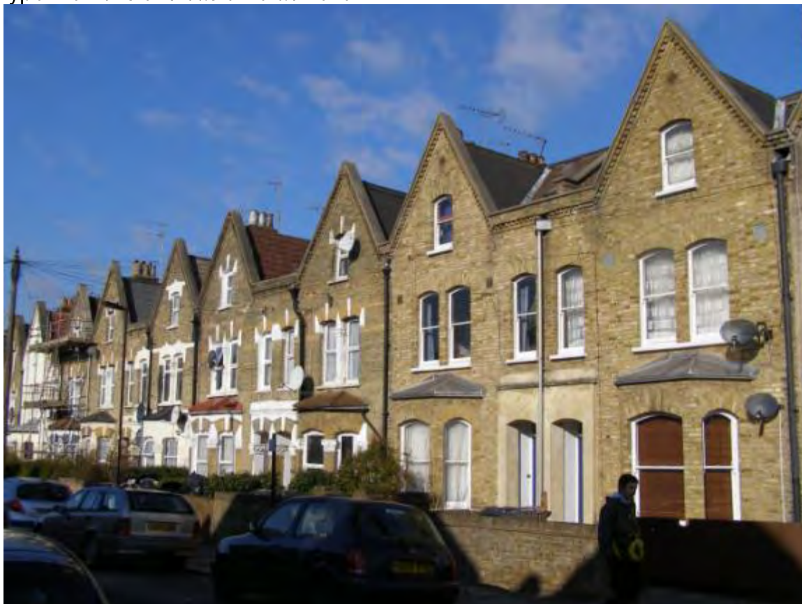
Figure 9; typical gable fronted terrace not suited to Type 2 and 3 extensions
