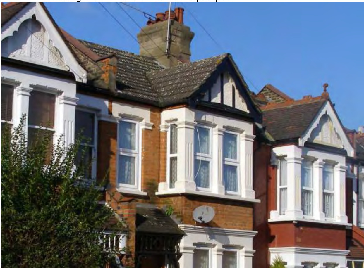
Figure 13 above:- Good example of existing decorative window surrounds; if any houses like these were extended, they should reproduce these details around the new windows. These mouldings would also form a good model for the decorative parapet to a “Type 2” extension
