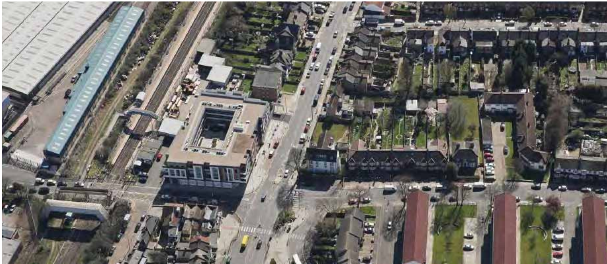
Figure 17 (top): Northumberland Park Station, view from North (Bing Maps)
