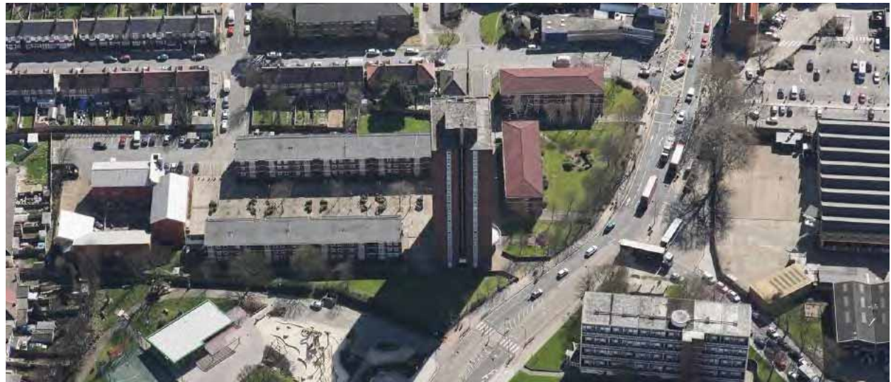
Figure 16 (below): Stellar House estate, view from North (Bing Maps)
