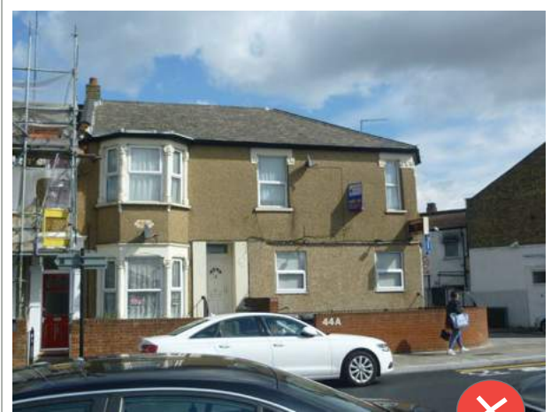
Brickwork should not be painted or covered with render, pebble-dash or cladding.
