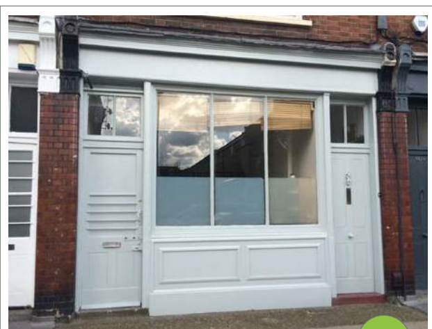
Original shop front features should usually be retained and adapted.
