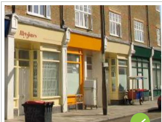
Internal shutters which don't obscure architectural features
