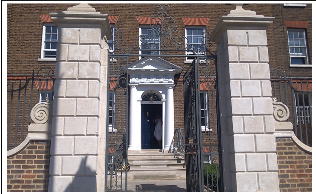
Entrance to Percy House, 796 High Road
