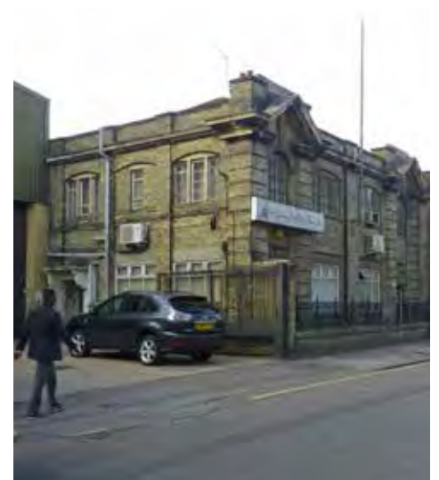
Employment buildings with historic and townscape merit along Ashley Road
