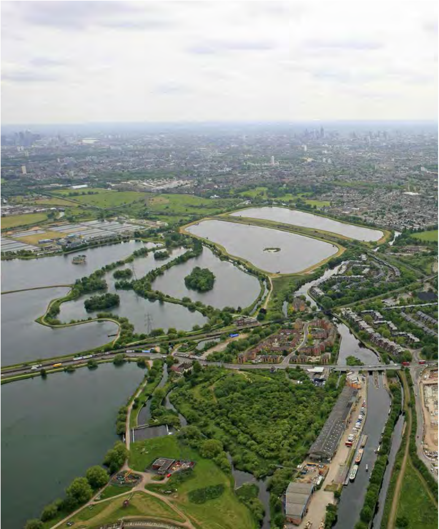
Aerial view of Hale Wgarf looking south
