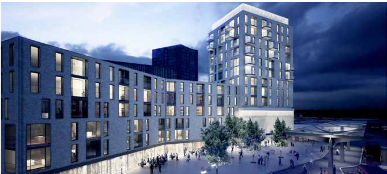
Tottenham Hale Station
