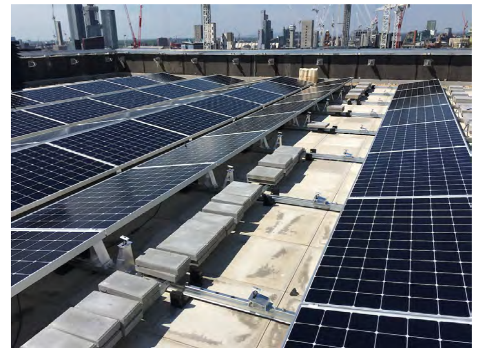
Figure 16 - Roof-mounted PV installations will have to be maximised. The panels selected should be high output and the concertina arrangement makes the most of the roof space available
