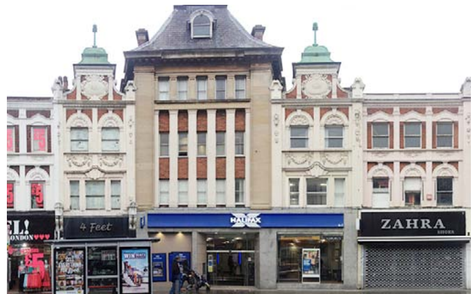
A2 - Halifax Bank within the former Empire Theatre
