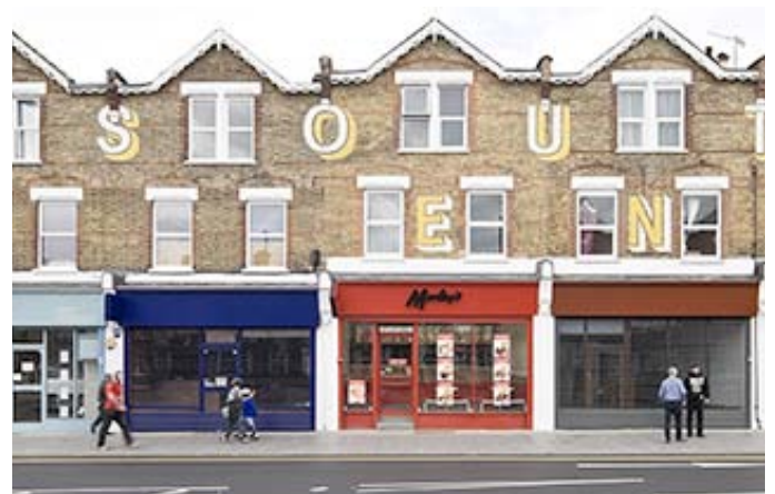
South End Activation, high street improvements by Hassell Studio
