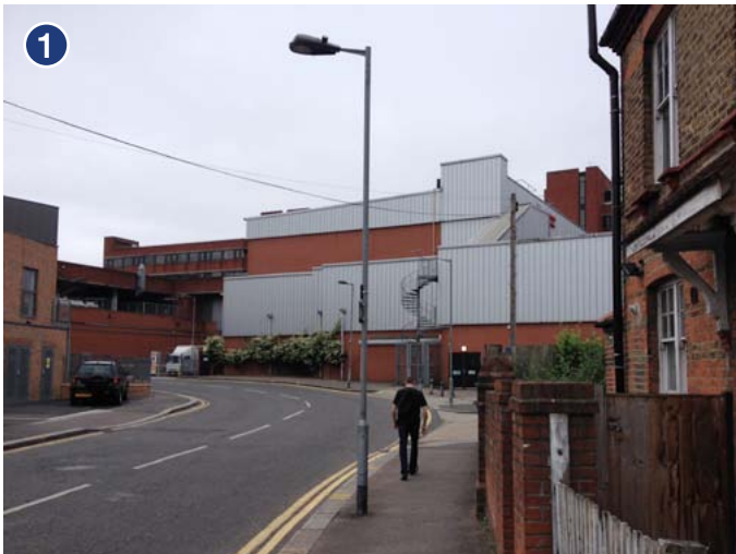
Service yards to the rear of the Mall
