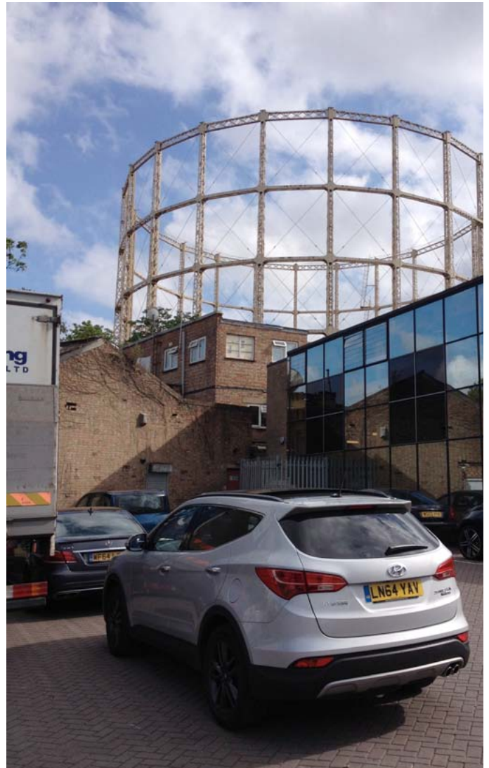
View of the gasholders from Bittern Place
