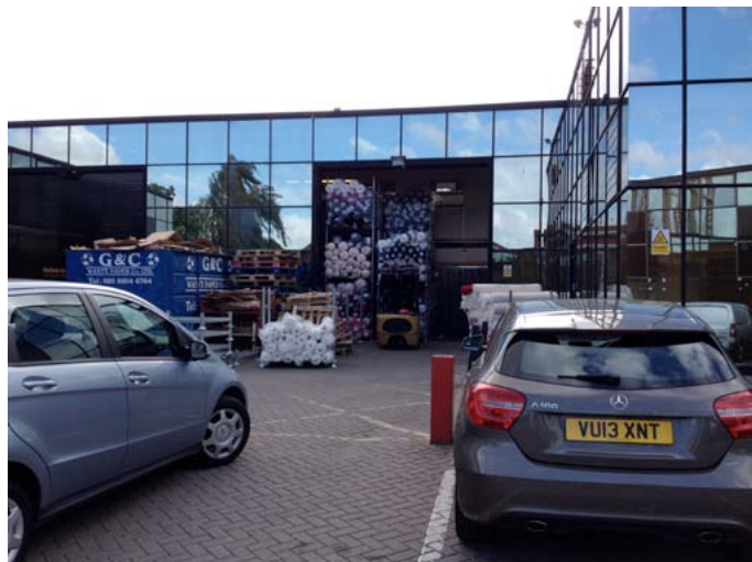
Industrial units and loading space within Bittern Place
